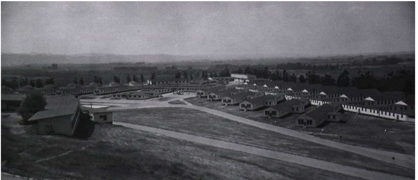
U.S. Naval Hospital, Corona, CA: General view of Unit III
